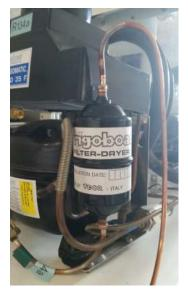
The filter drier works correctly in the vertical position with the arrow indicating direction of flow as shown in the enclosed photo. Filter drier should be secured with copper pipe not chafing or vibrating.
